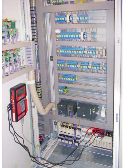
Control cabinet with an eTracker measuring instrument connected up
