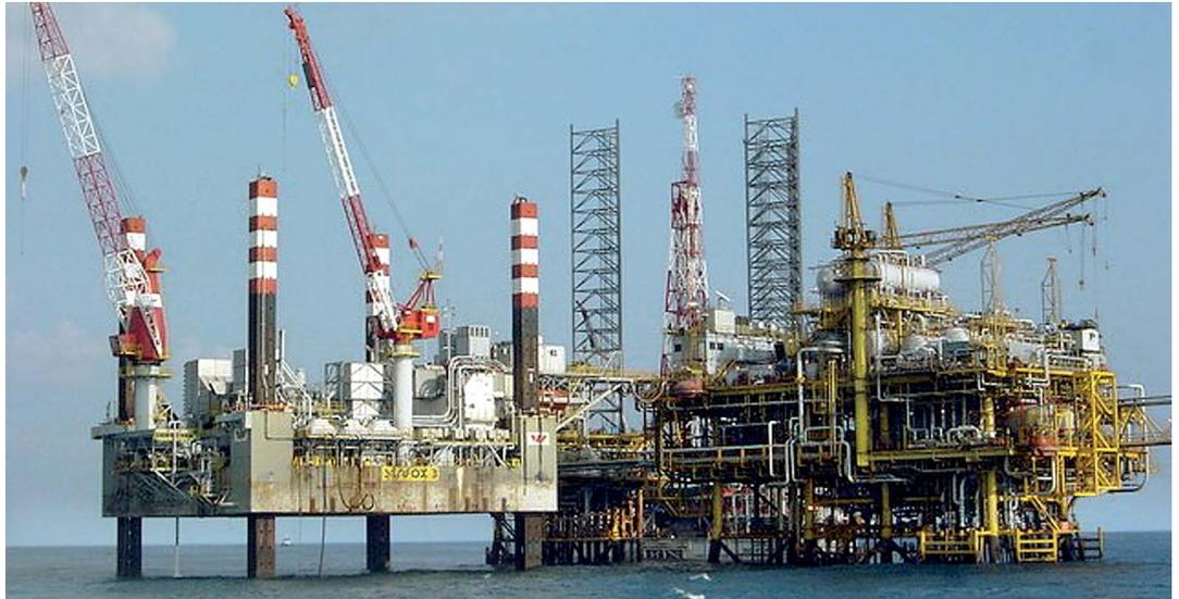
Seafox platform, Indonesia, operated by the Chinese National Offshore Oil Cooperation, equipped with Viledon T 60 and T 90 pocket filters in the air intakes of gas turbines
